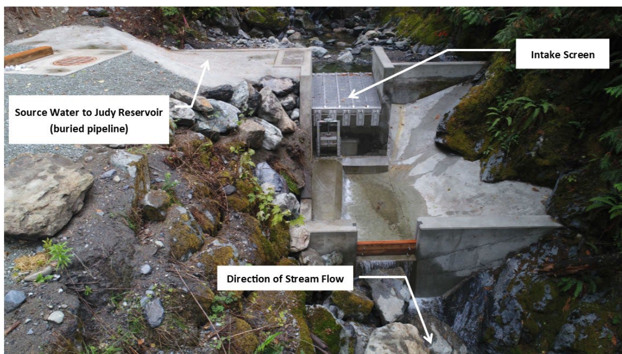
Figure 2-11. Mundt Creek Diversion
