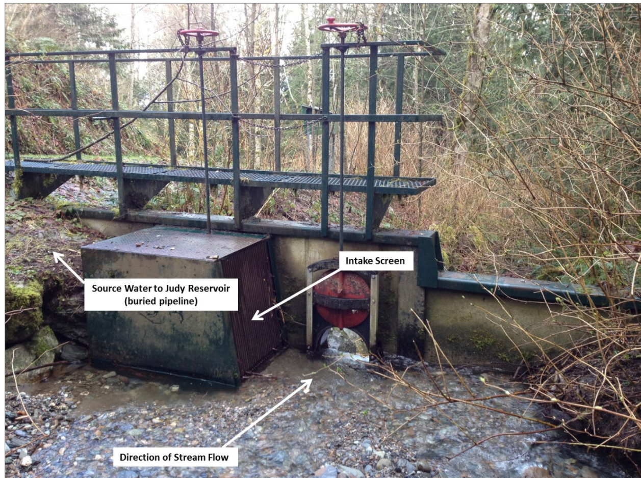
Figure 2-13. Salmon Creek Diversion
