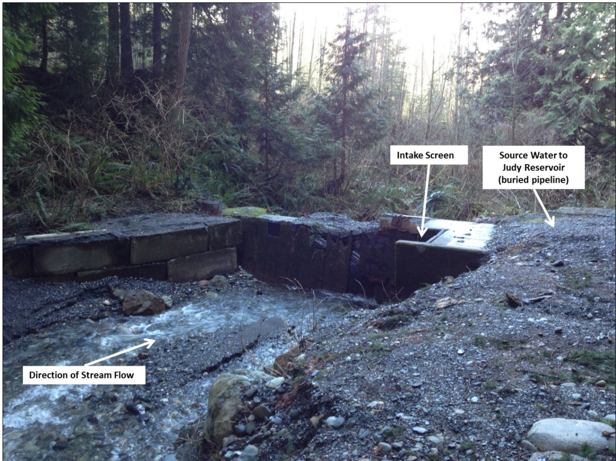
Figure 2-12. Turner Creek Diversion
